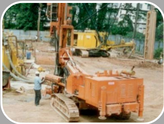
Singapore - Pre-Bored H Pile Ø560 mm
