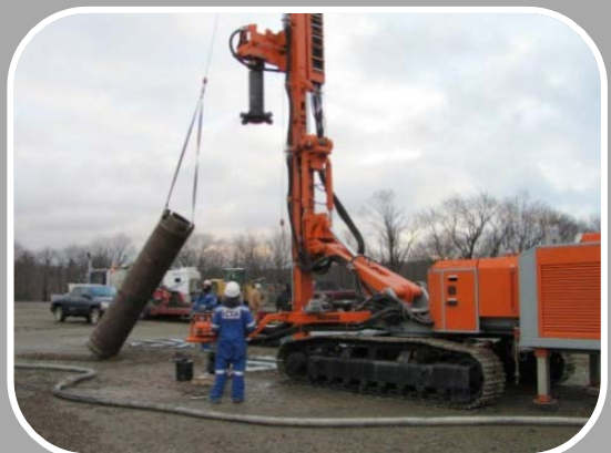
USA - DTH Hammer Drilling Ø610 mm
