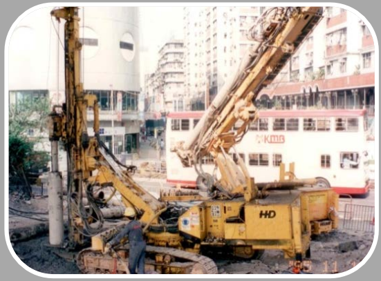
Hong Kong - DTH Hammer Drilling Ø560 mm
