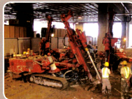
Hong Kong - Grout Hole Drilling \phi 101.6\text{mm} Hong Kong - Verpressbohrung \phi 101.6\text{mm}
