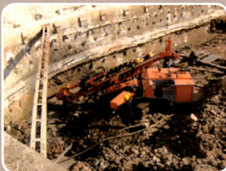
China - Anchor Drilling \phi 101.6\text{mm} China - Ankerbohren \phi 101.6\text{mm}
