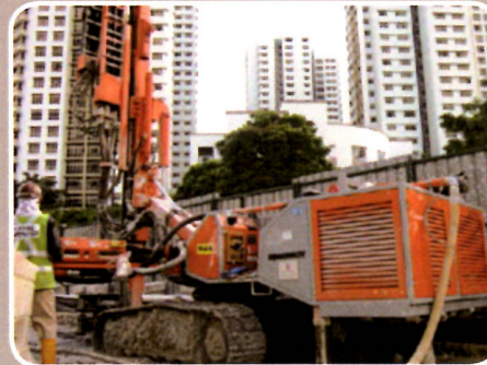
Singapore - Grout Hole Drilling \phi 88.9\text{mm} Singapore - Verpressbohrung \phi 88.9\text{mm}
